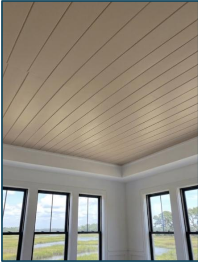
Owner's Suite: 1x6 Painted V-groove in tray ceiling
