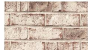
BRICK & MORTAR – OLD EDISTO WITH WHITE MORTAR
