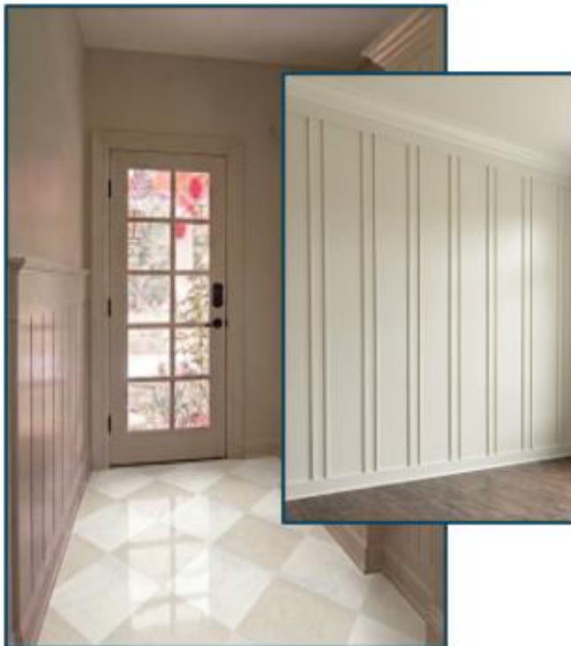
Mudroom: Board & Batten Wainscot Along Left Wall Using With 1x6 Hook Rail & Cap
