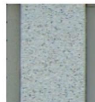
Stucco Foundation: Tabby Shell Mix with Holcim Old Lime Putty Mortar
