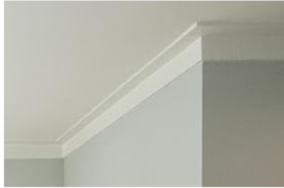
CRAFTSMAN CROWN (1x4 on ceiling with 1x6 wall plate)
